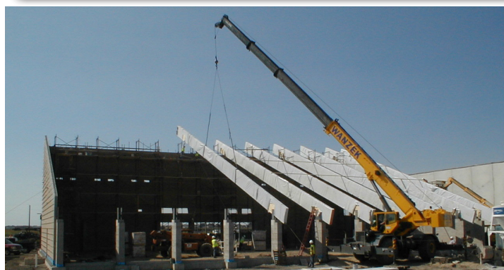
Placing the beams for the Sanctuary
