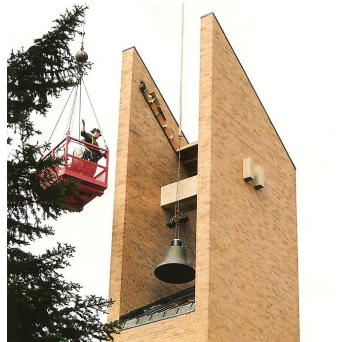
Hanging the bell at the original church—the same bell that now hangs in the current bell tower.
